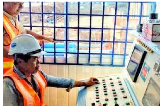
Computer guidance systems for pipe jacking
