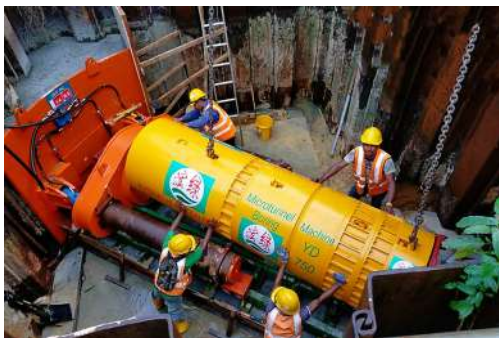
Jacking machine and thrust pit setting up
